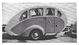
Using only hand tools. Monte La Flecke built this sportsmantype trailer. It is 113/4 feet long and sleeps two comfortably.
