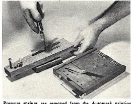
Pressure springs are removed from the Automask printing frame and screwed to the wood lever.
