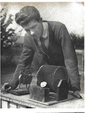
Above — The recording thermometer in operation. The lines scratched on the cylinder are visible on the right side.
