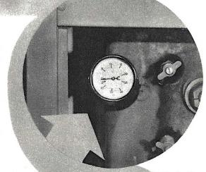
Above—This is type of double reading gauge which should be used with vacuumized heating system. Below—Water gauge fittings should be repacked to eliminate possibility of air leaks.
