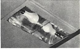
The top photograph shows the reflector completed and ready to be installed into the ceiling. Below—The lights in place and ready to supply ample illumination for Ping Pong table.
