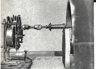
Top—The detailed drawing shows the method of hooking up the cylinder to the clock motor. Although a universal joint is used, the builder should attempt to line up the two shafts as correctly as possible. Above—The recording cylinder hooked up to the motor with its outside case removed.
