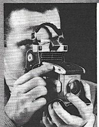
The photoelectric cell, mounted behind multiple collective lenses, automatically preselects proper aperture for the picture.
