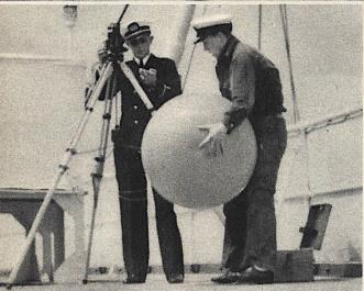
Above—Many ships serve as weather stations for the ocean-flying lines, sending aloft balloons to determine, by theodo-lite recordings, the wind speed and direction at various alti-tudes, the information being radioed to flight stations ashore.
