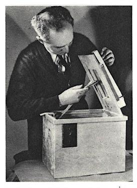
The top of the printer may be raised for "local control" or to give additional exposure to any part of the print with a concentrated beam of light, such as obtained from a "pen light" flashlight.
