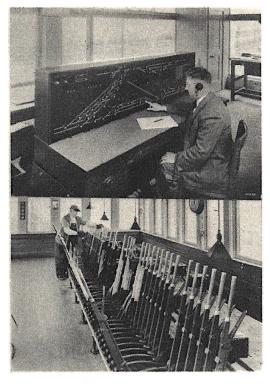
ELECTRIC trains crossing the San Francisco-Oakland Bay Bridge operate under a modern electric interlocking and signal system which is actuated by a push-button control board only 6½ feet long (top). A mechanical lever system of similar capacity (lower) would require 60 feet of space.
